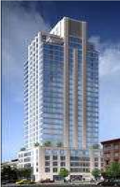
450 EAST 83 RD STREET
